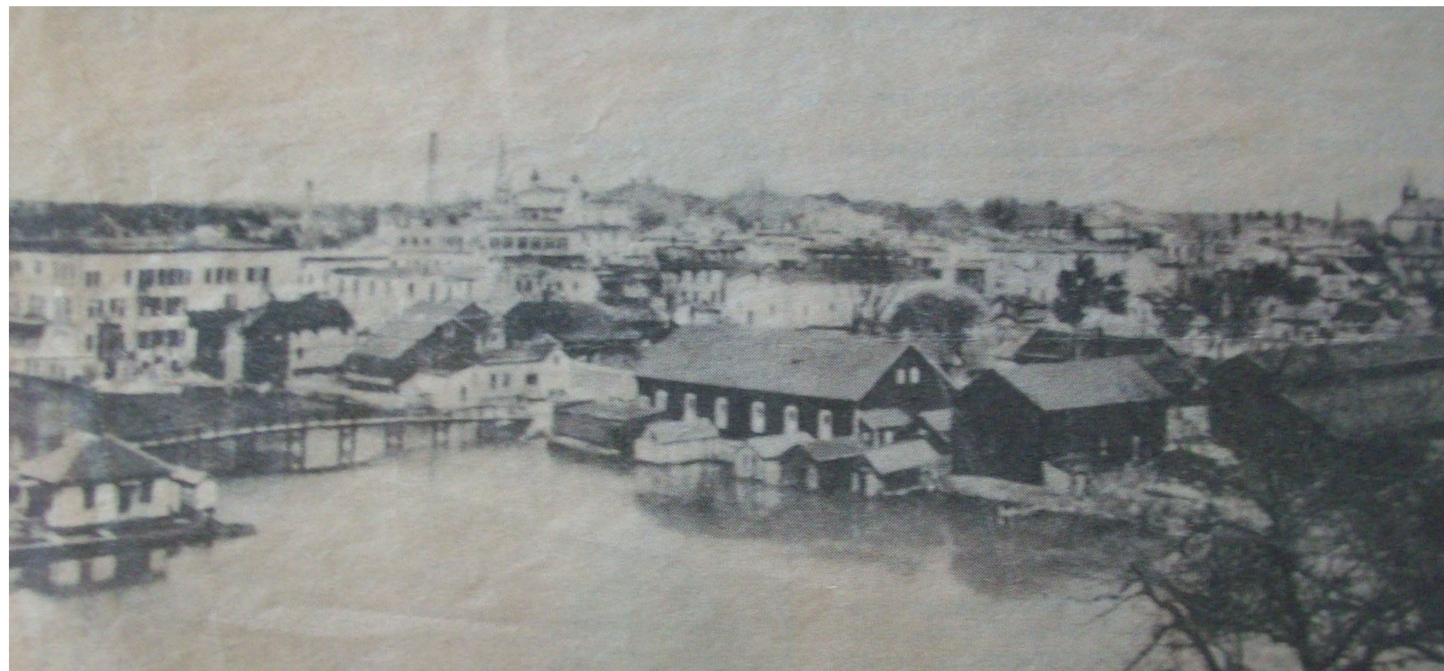
Jefferson Street walkbridge, Stoughton, WI, 1909. Courtesy Stoughton Historical Society
