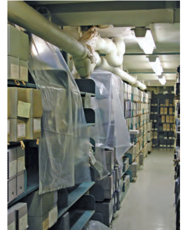
Overhead water pipes above archival storage boxes illustrate a clear preservation need
