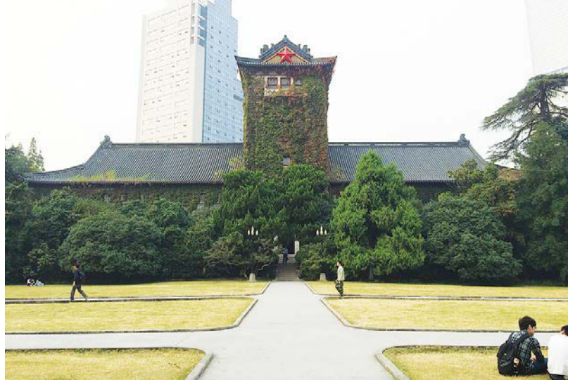
Nanjing Administration building (October 2014).
