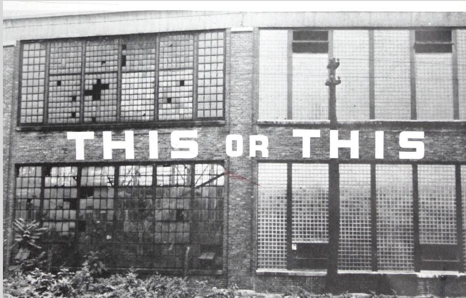
Owens-Illinois Glass Company promotional image showing the benefits of replacing metal industrial sash with glass block. Source: Owens-Illinois Glass Company, Insulux: Subject Heating...Answer, Insulux Glass Block (Owens-Illinois Glass Company, 1941), http://archive.org/details/InsuluxSubjectHeating...AnswerInsuluxGlassBlock , 1.
