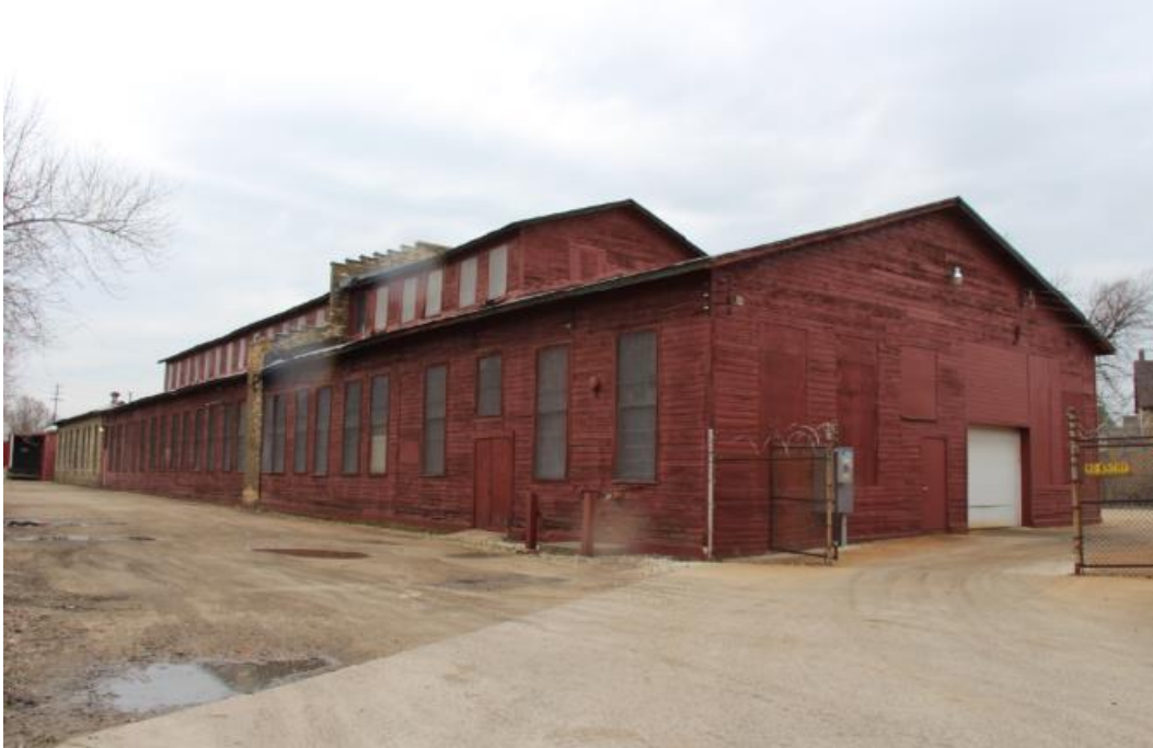
Figure 29. Milwaukee Hay Tool Company factory, 2773 S. 29 th Street, view facing northwest.
