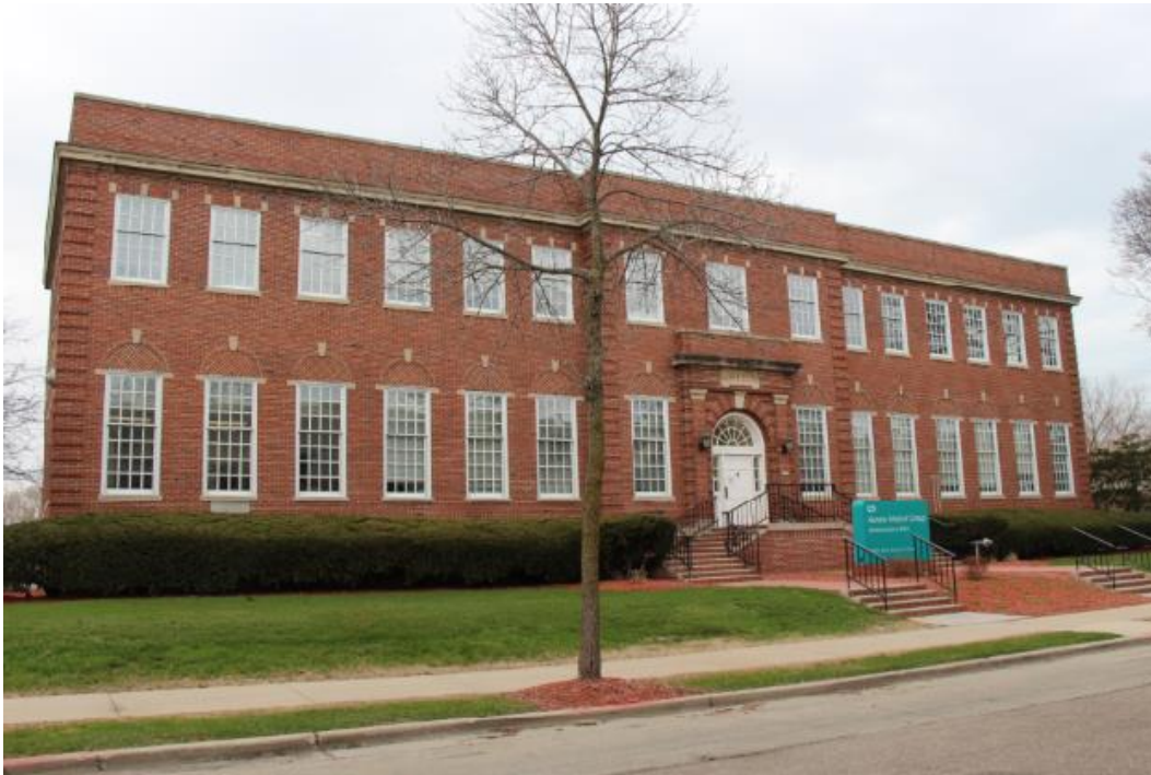
Figure 30. Heil Company Office, 3000 W. Montana Street, view facing north.
