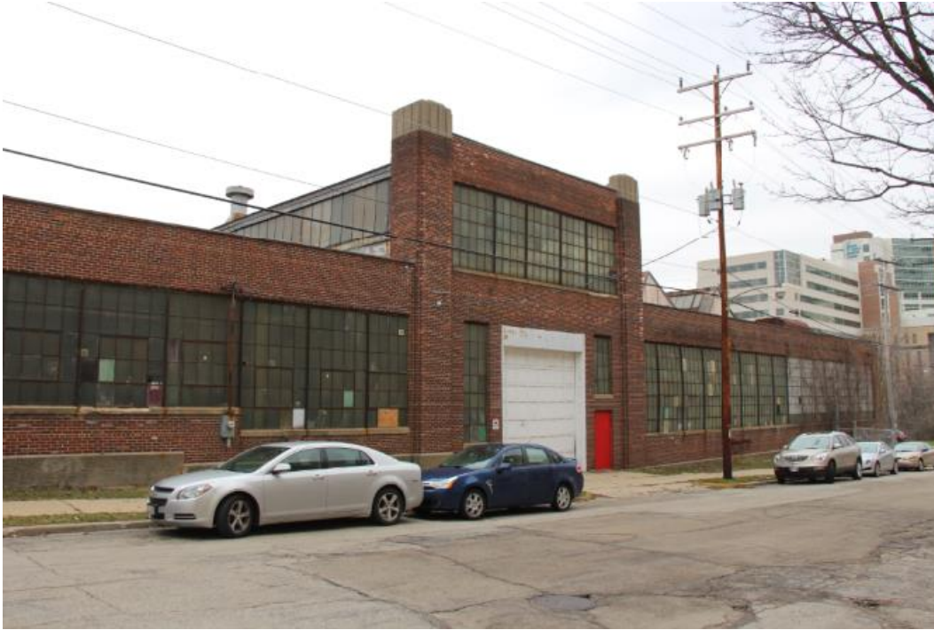
Figure 31. Heil Company factory, 2844 S. 29 th Street, view facing southeast.
