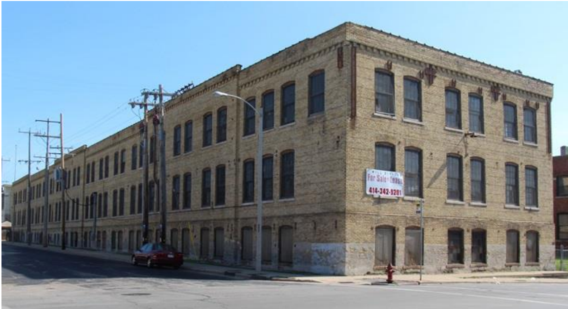
Figure 13. This c.1900 industrial loft housed a portion of the Romadka Brothers' Co. suitcase factory, later part of Briggs & Stratton's West Side plant (AHI No. 111593, 2748 N. 32 nd Street). Staining, varnishing, and blacksmithing departments were located at ground level, with the main factory floor above and warehousing on the uppermost level. 107
