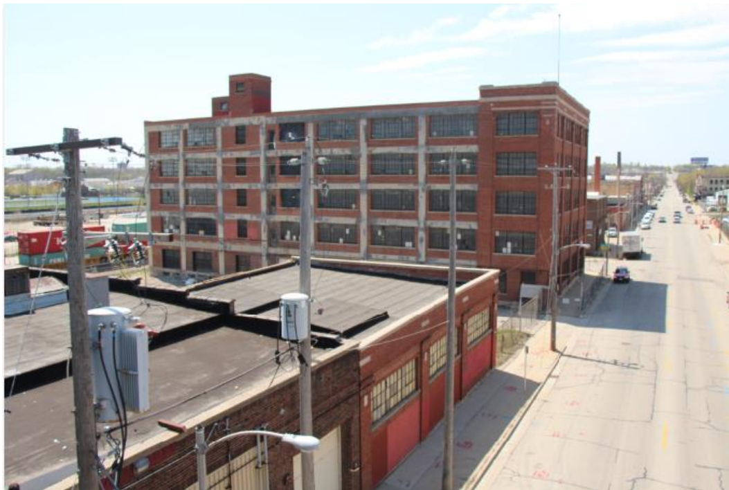
Figure 33. View along W. St. Paul Avenue from 16 th Street viaduct, facing southwest.
