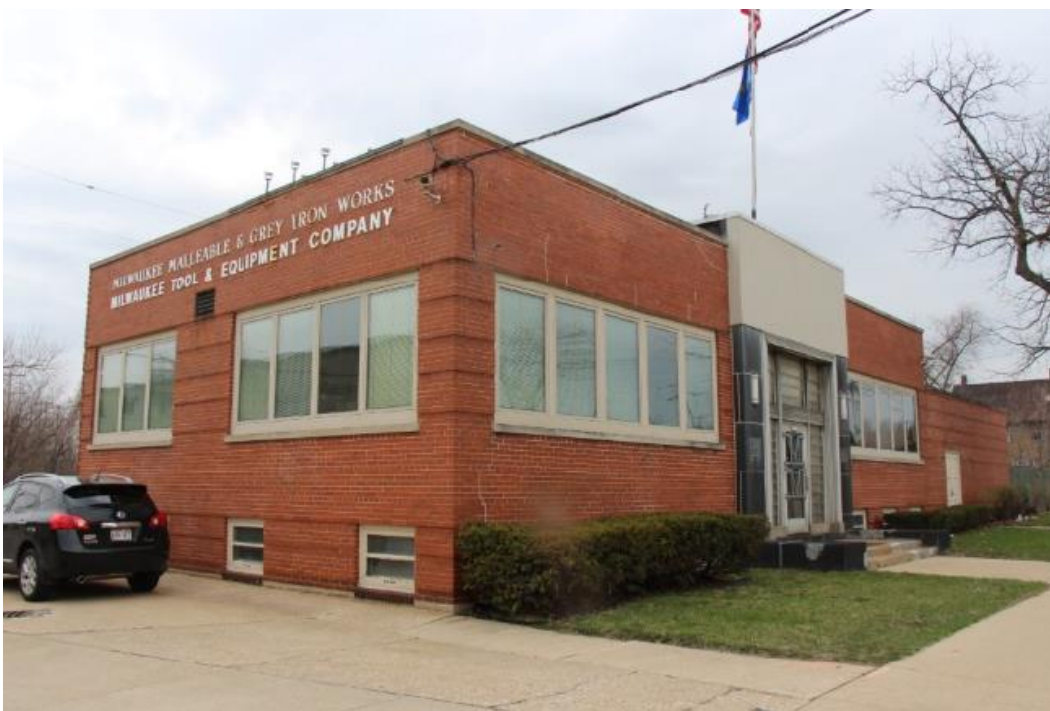
Figure 28. Milwaukee Malleable and Milwaukee Tool Company office, 2773 S. 29 th Street, view facing northwest.
