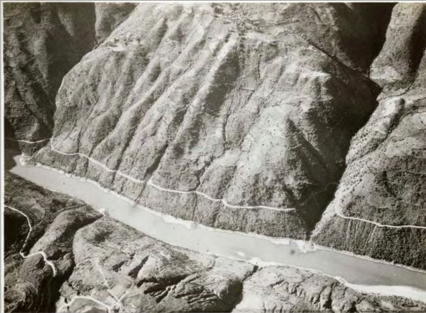
AERIAL VIEW OF A PART OF THE LEDO-BURMA ROAD. 28 JAN. 1945.
