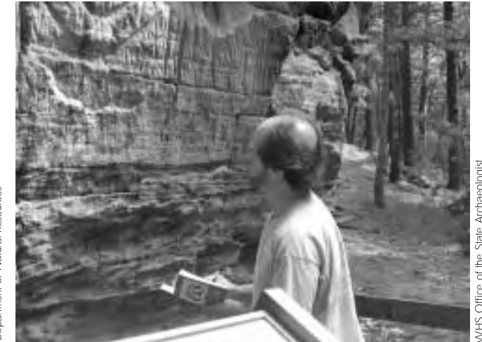
State Archaeologist John Broihahn assesses recent damage to the Roche-A-Cri site.
