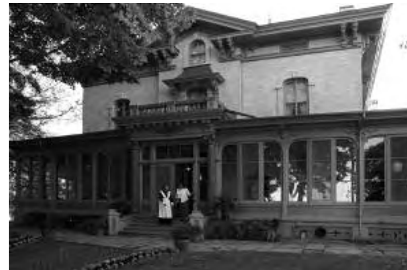
The grand Italianate exterior of Villa Louis, which was constructed in 1870-1871 and designated a National Historic Landmark in 1960.
