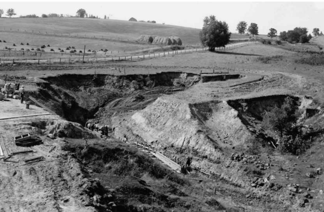
CCC crew installing a drainage canal in Vernon County to control erosion, 1937. Enrollees from the Soil Conservation Service camp at La Valle were doing the same work at the same time on farms in Sauk County.
