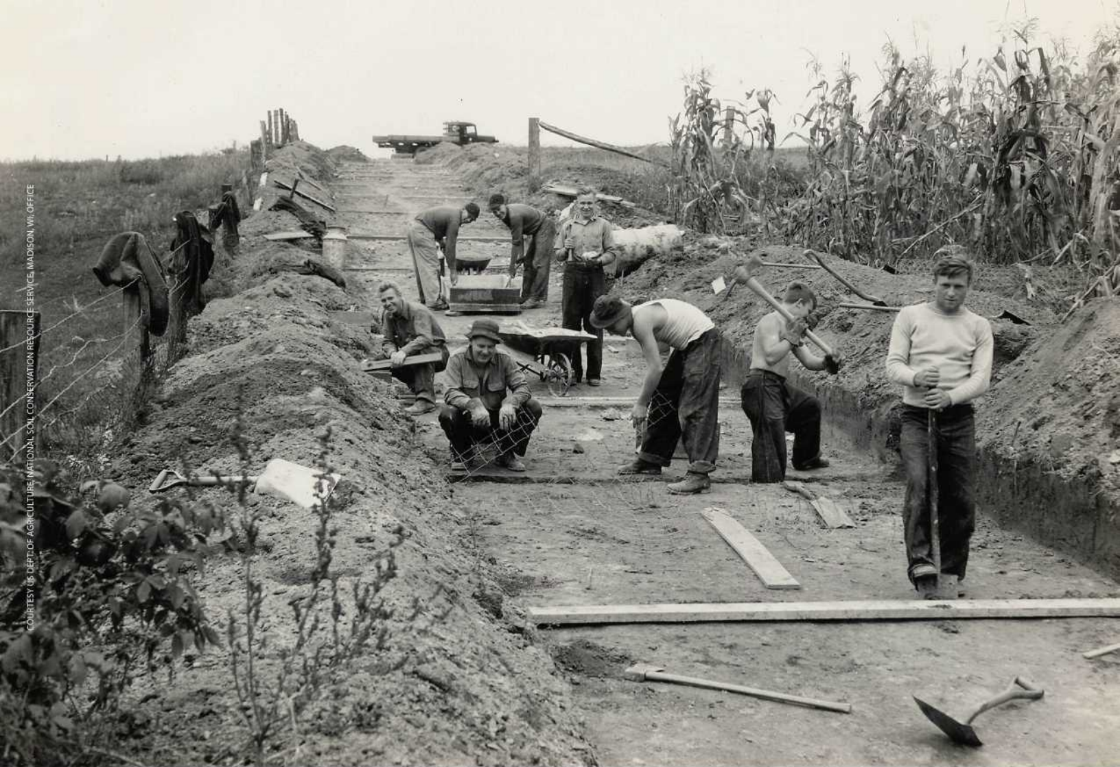
This 1934 terrace outlet project from Coon Valley, Wisconsin, is designed to channel water down a hillside while protecting cropland from soil erosion. The La Valle camp enrollees engaged in identical work in Sauk County.
