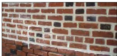
Example of mismatched mortar
