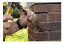
To remove deteriorated mortar properly, hand chiseling is the method least likely to cause damage to the
