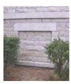
should match those of the wall and should be inset from the face of the wall at least two inches. Non-original windows can usually be closed flush to the wall surfaces with matching materials.
